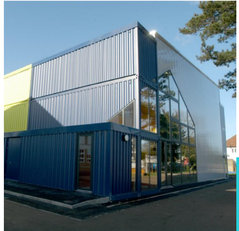
BCIA Awards- Small Building of the Year Dunraven School Sports Hall commended for the reuse of shipping containers
